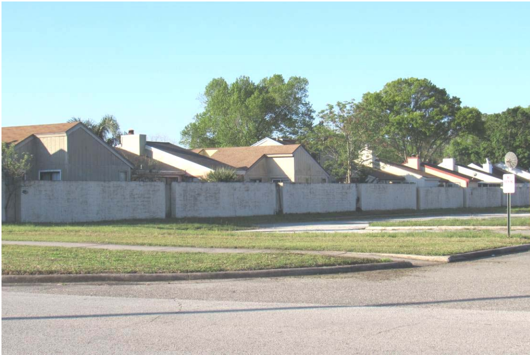
View of existing 6 foot high masonry wall adjacent to single family and duplex dwellings.
