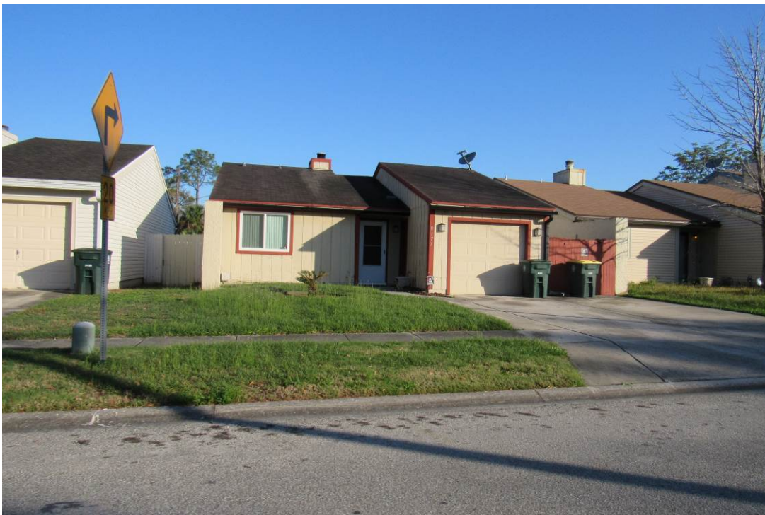
Existing duplex adjacent to proposed development.
